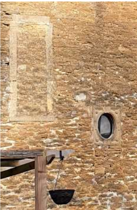
The northern flank wall of no. 18 Pickwick features a delightful decorated window frame and a blocked-up window
