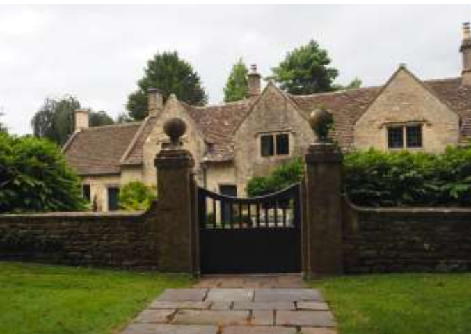
Missing window mullions above and below. There would have been two mullions per window in the building shown below (evidenced by the window head joints).
