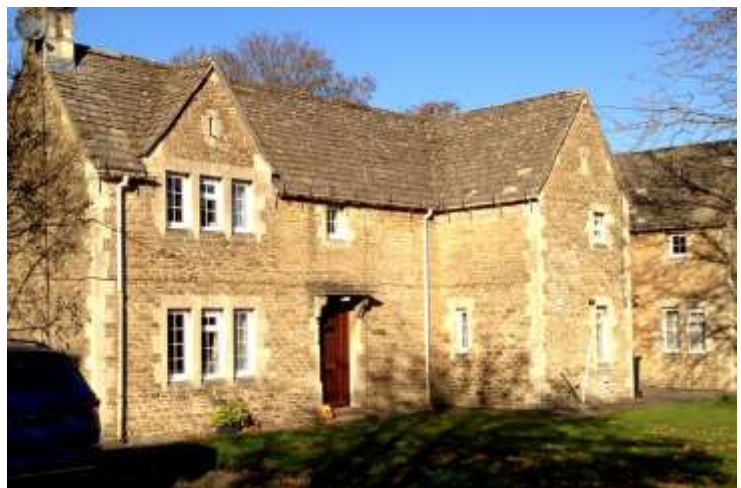
Interwar artificial stone tiling at Hudswell
