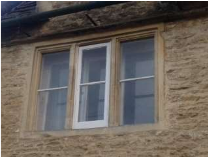
Mullioned window—iron casement replaced by new softwood
