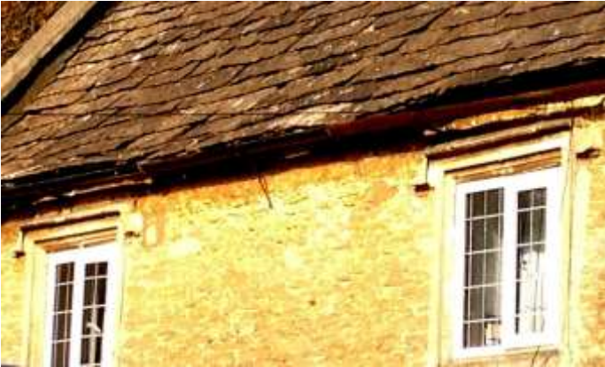
Missing window mullions above and below. There would have been two mullions per window in the building shown below (evidenced by the window head joints).
