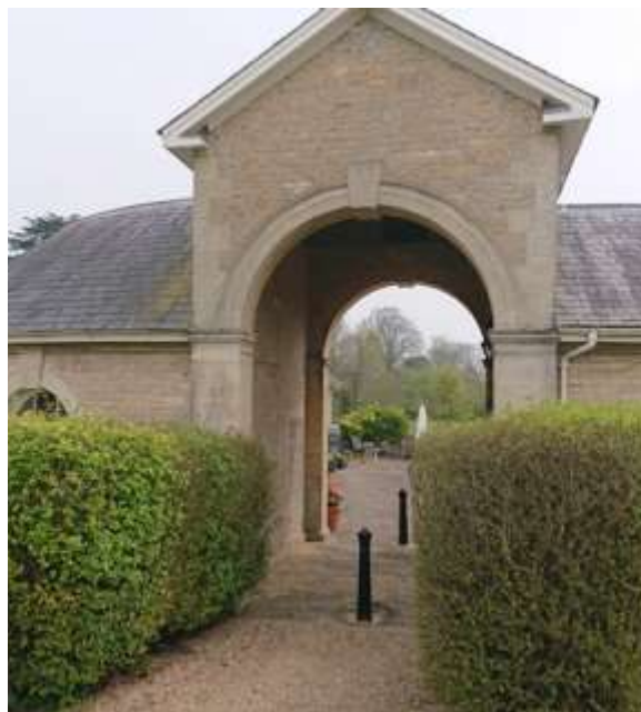
The arch through the Stables at Beechfield
