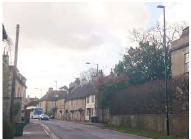
Three different design street lights in 100 yards
