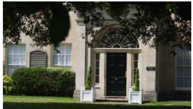
Main entrance to Beechfield House featuring a decorated semi-circular fanlight typical of fine houses of the period
