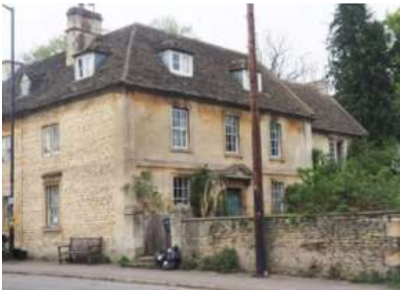
Below: Nos 41,41a, the Masonic Hall, Nos 43 and 45
