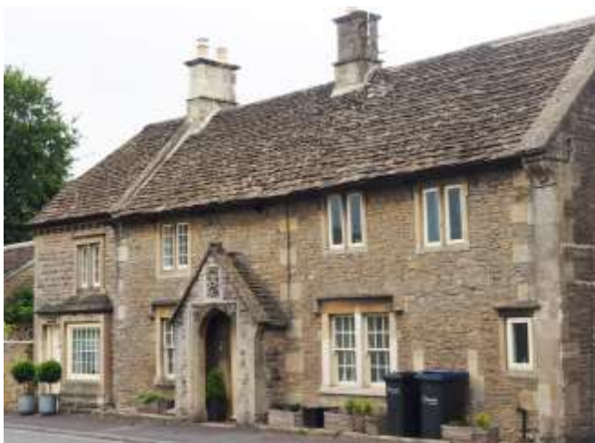
Poynder porch added to older house
