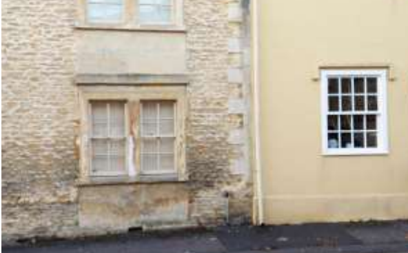
Above - Artificial stone quoins in Corsham
