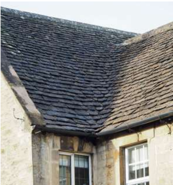
Swept stone tile valley, above; cut stone tile valley, below
