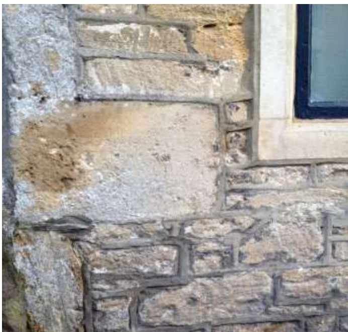
Cement rich ribbon pointing in Pickwick Street
