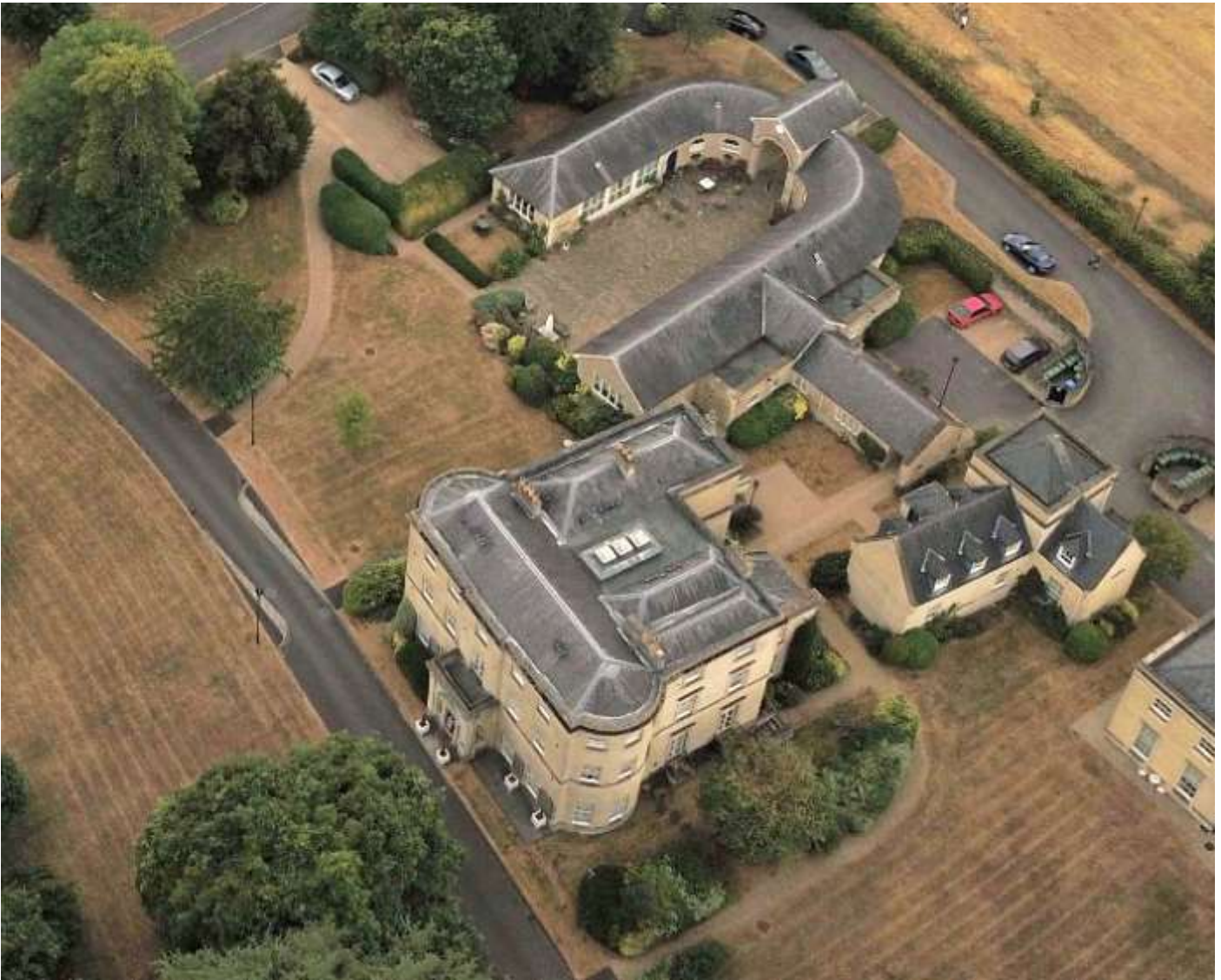
Beechfield House and The Stables
